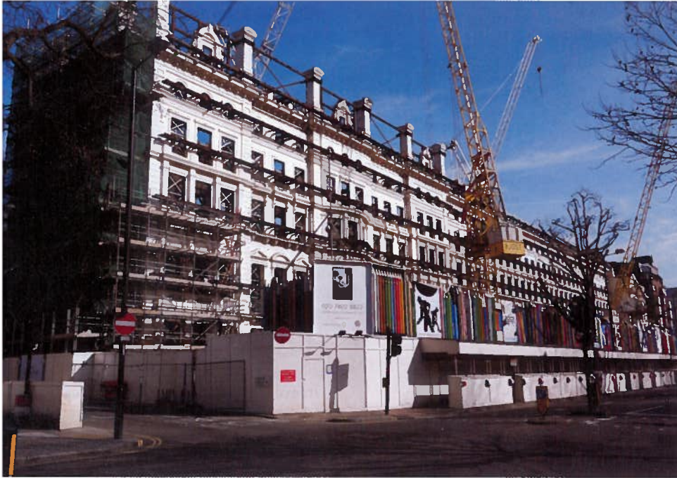
The refurbishment of this terrace reinstates it as one of London's most upmarket residential developments. It is the UK's largest ever retained facade
